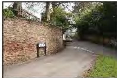
High walls (of sandstone and mortar slates) define property boundaries.
